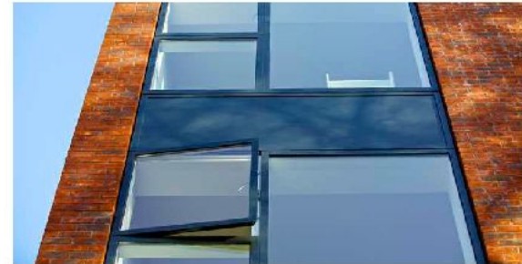
INDICATION OF TYPICAL ALUMINIUM TIMBER COMPOSITE WINDOWS AND PANELS BUT WITH PROPOSED COLOUR - RAL 7012 BASALT GREY
